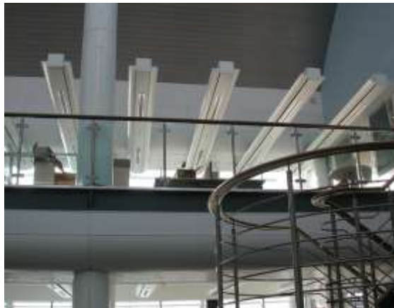
Devonshire Building, Newcastle
