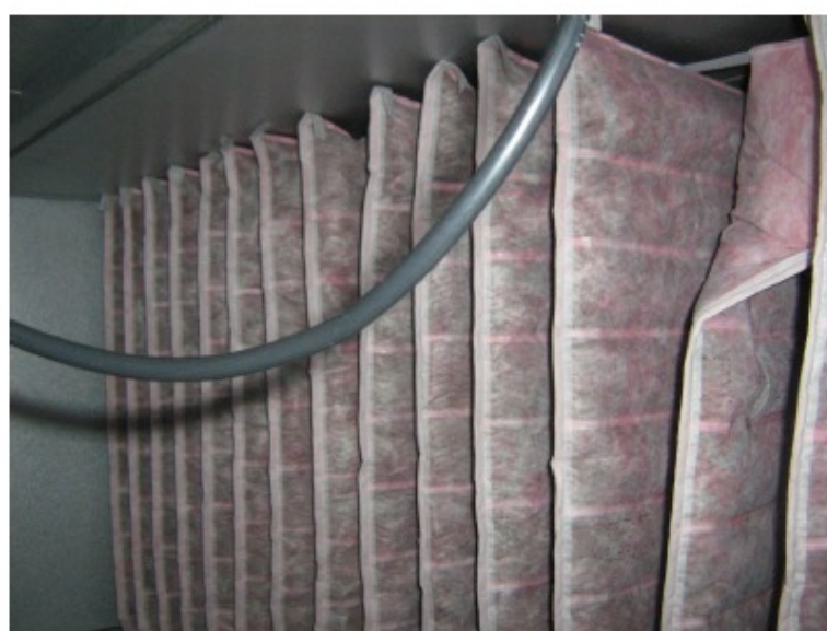
Same filter package, after three months use 24.1.2011. Surface absolutely dry, the darker colour is due to soot on the filter surface.
